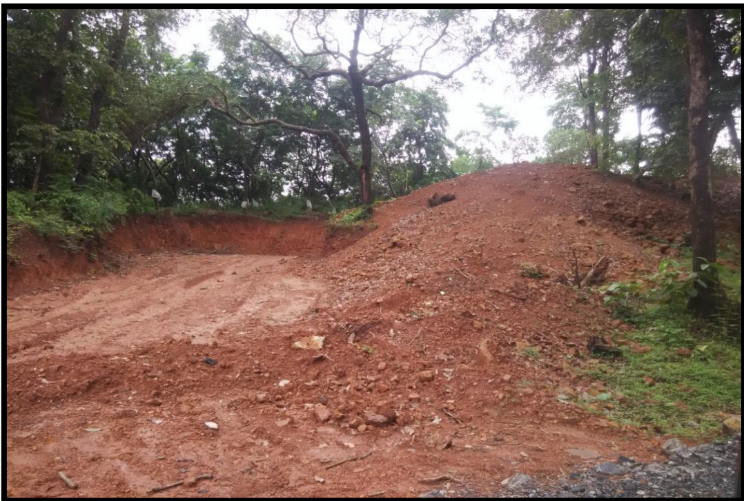
Top soil stacked in project site
