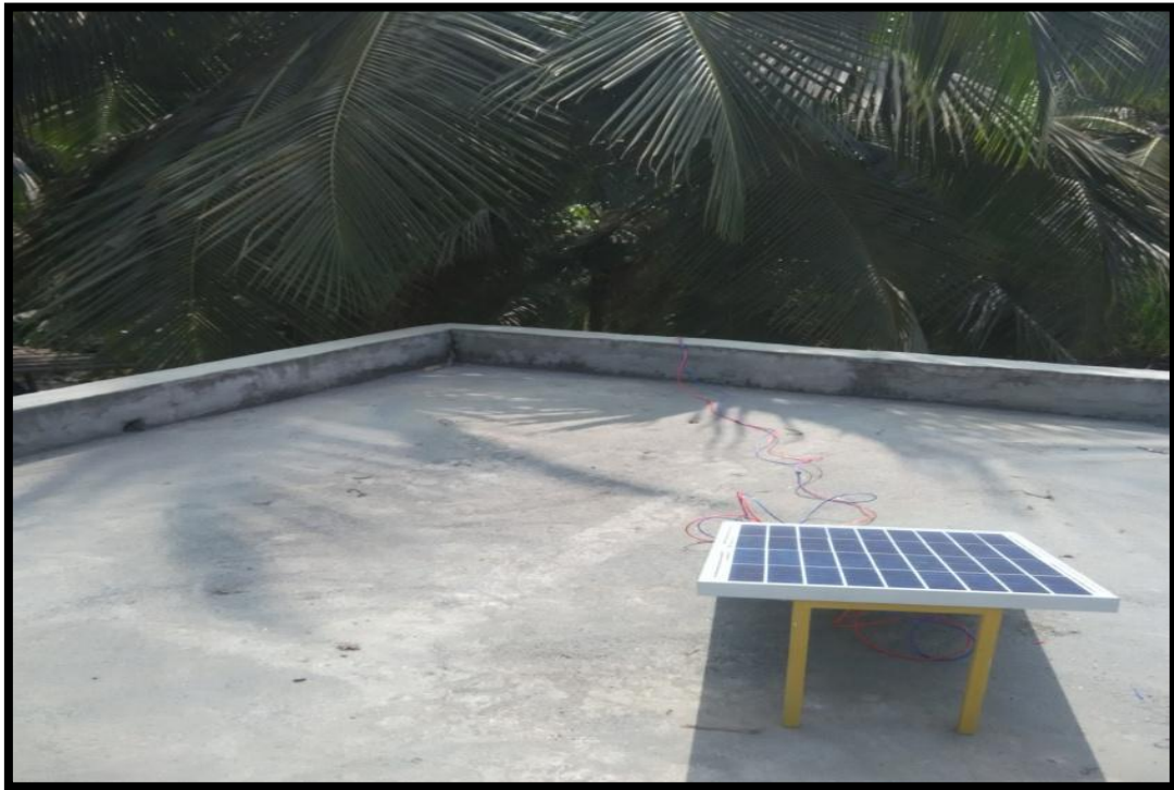
Solar panel installed in project site
