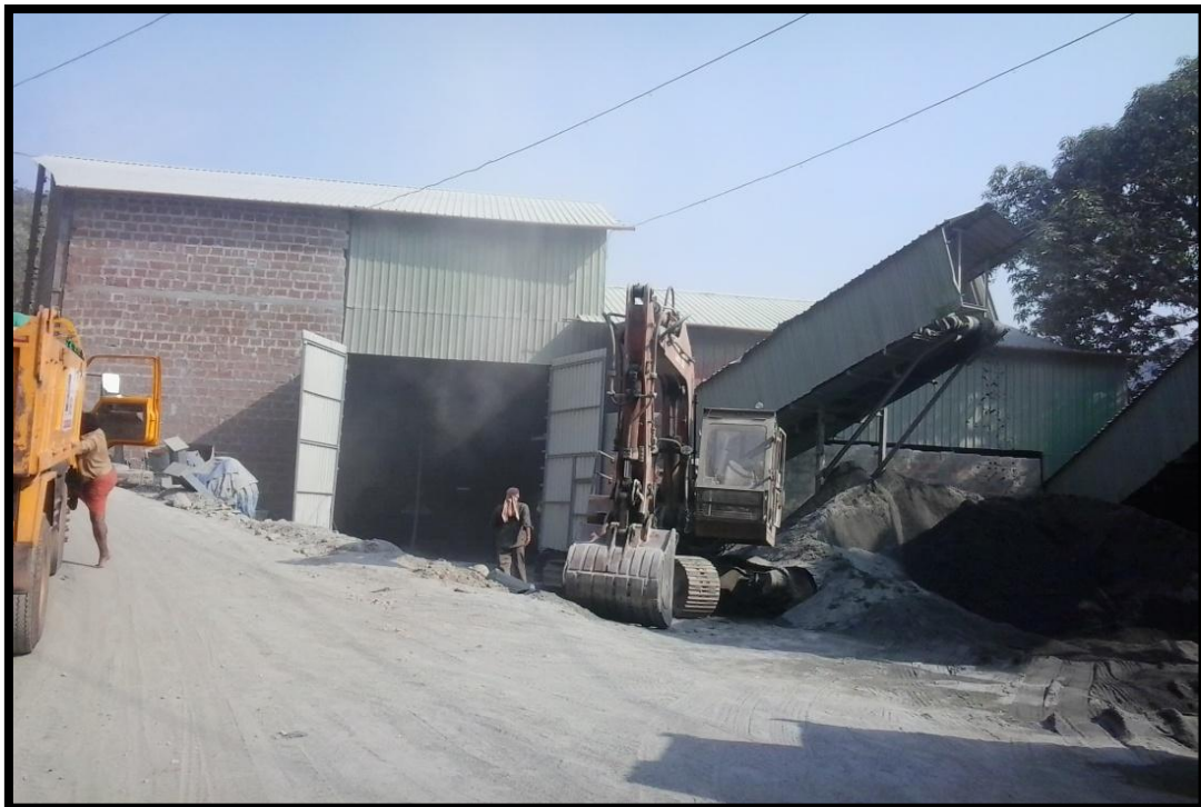
Crusher in the project land
