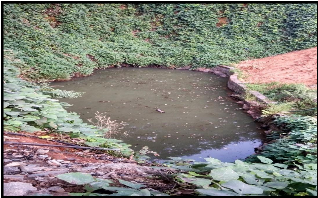
Rain water Collection pond – I
