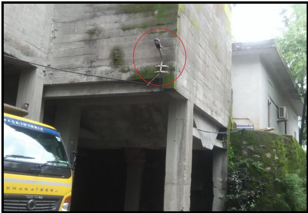
Solar Street Light
