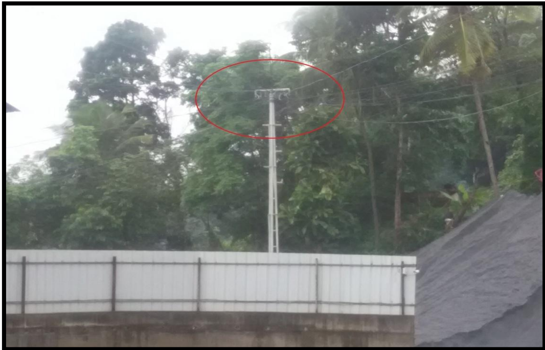
Sprinklers installed in the project area
