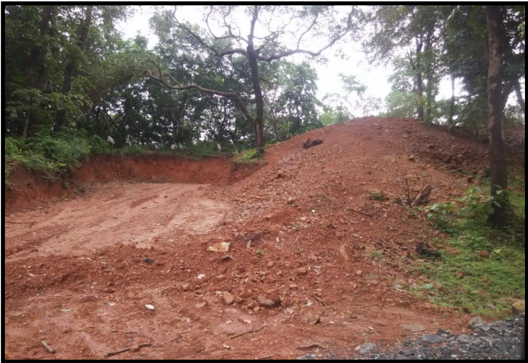
Top soil stacked in project site
