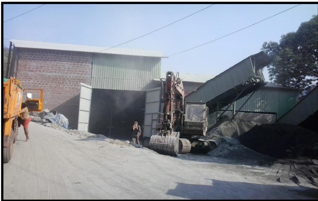
Crusher in the project land
