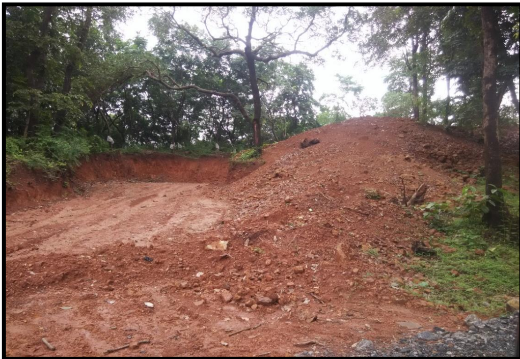
Top soil stacked in project site
