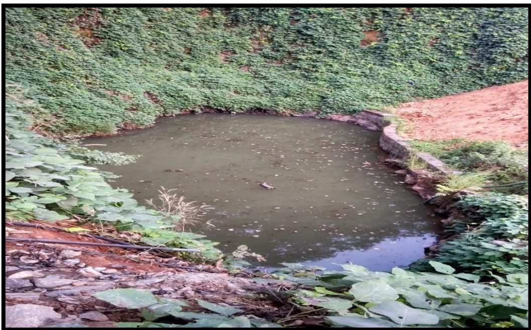
Rain water Collection pond – I
